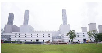
Beijing Thermal Power Plant's Gas Turbine Flue Gas Waste Heat Utilization Project
