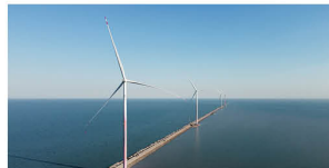
Tianjin Port Breakwater Wind Power Project
