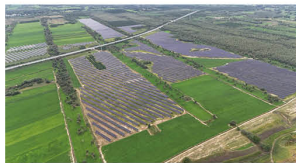
Zhangwu Photovoltaic Sand Control Demonstration Project
