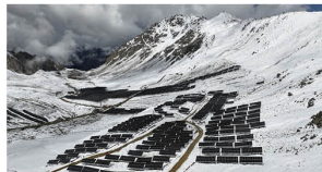
Phase I of Nagu Solar Power Station
