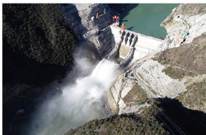
Wunonglong Hydropower Station
